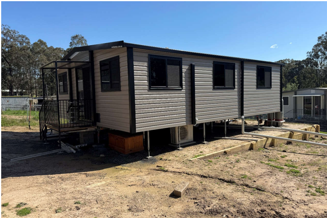
PHOTO 1 - SITE PHOTO LOOKING NORTHWEST
